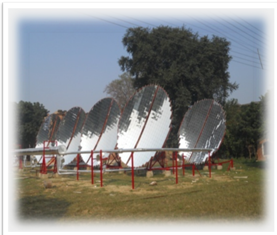
Fig 10 : Solar Thermal Cooking System at DEI Hostels
