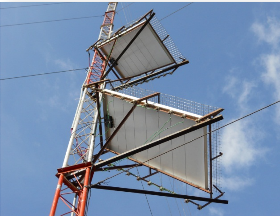
Fig 9 :Solar power for the radios of Wi-Fi tower with theft prevention measures in the forest region of Rajaborari, Madhya Pradesh
